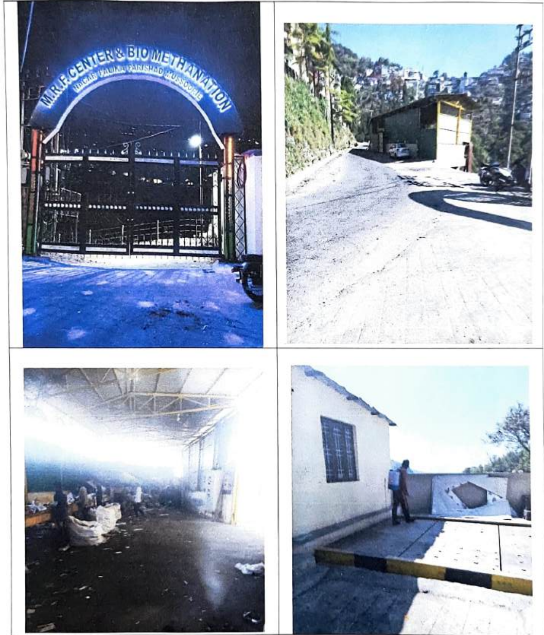
Photos of MRF Centre with Weighbridge
