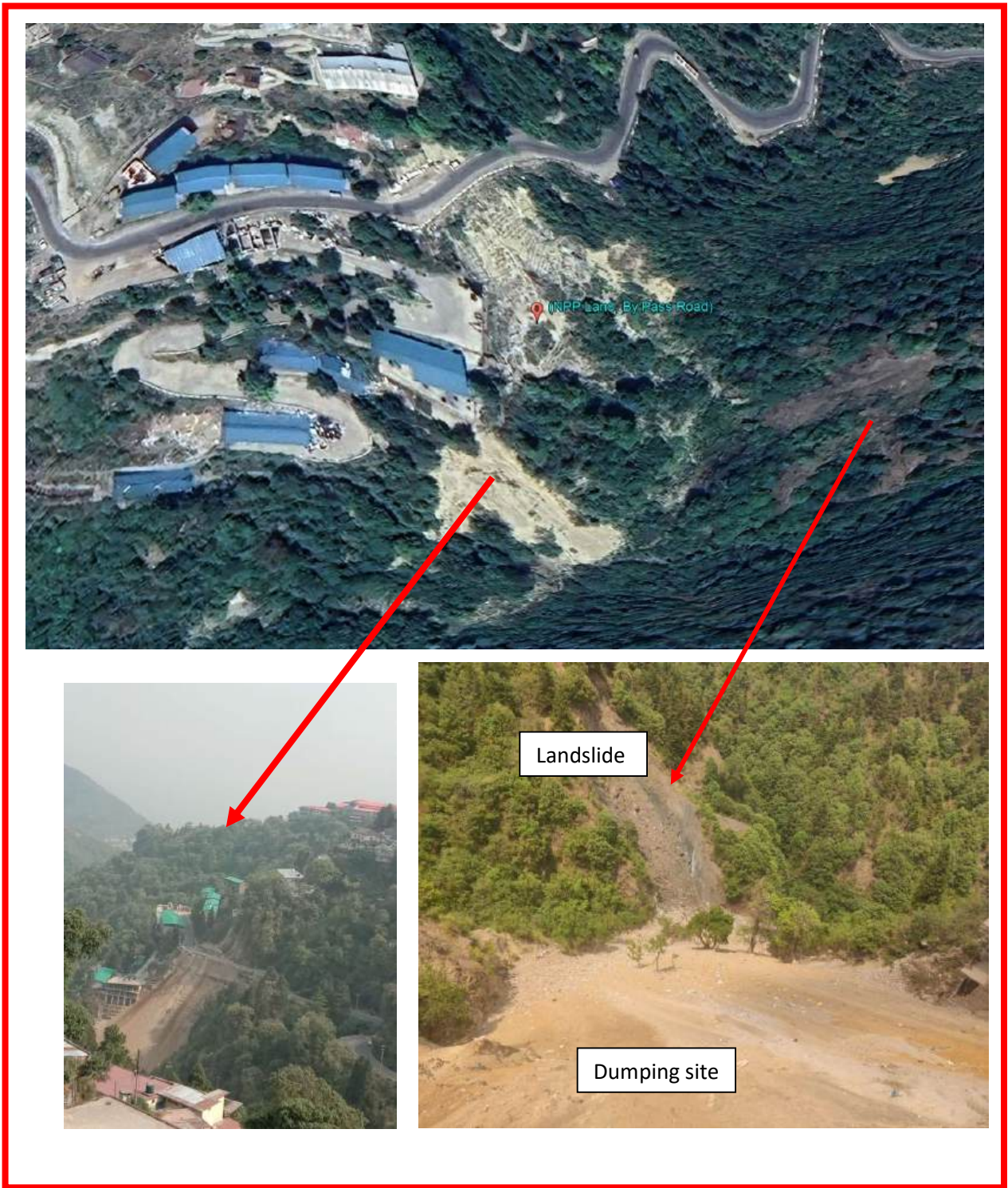
Figure 12 . Dumping Zone and Shallow landslide scarp present at site 8
