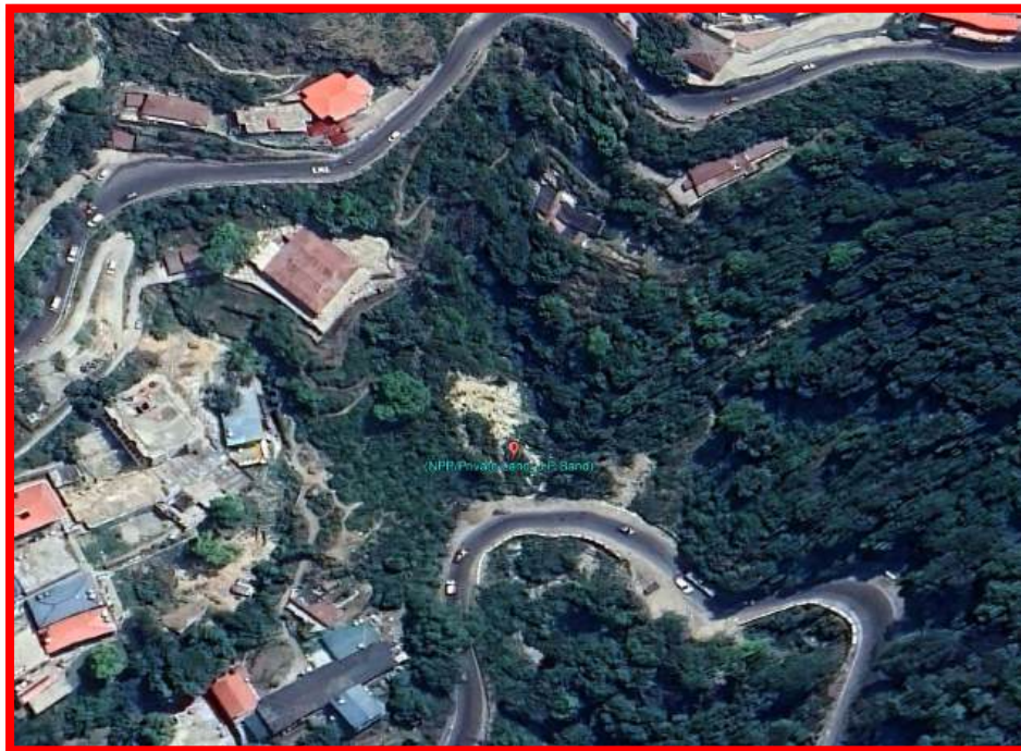
Figure 13 exhibiting the degrade slope along seasonal rivulet at site 9
