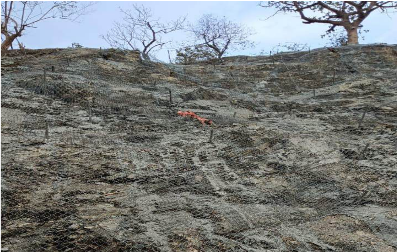
Installation of Chain link mesh
