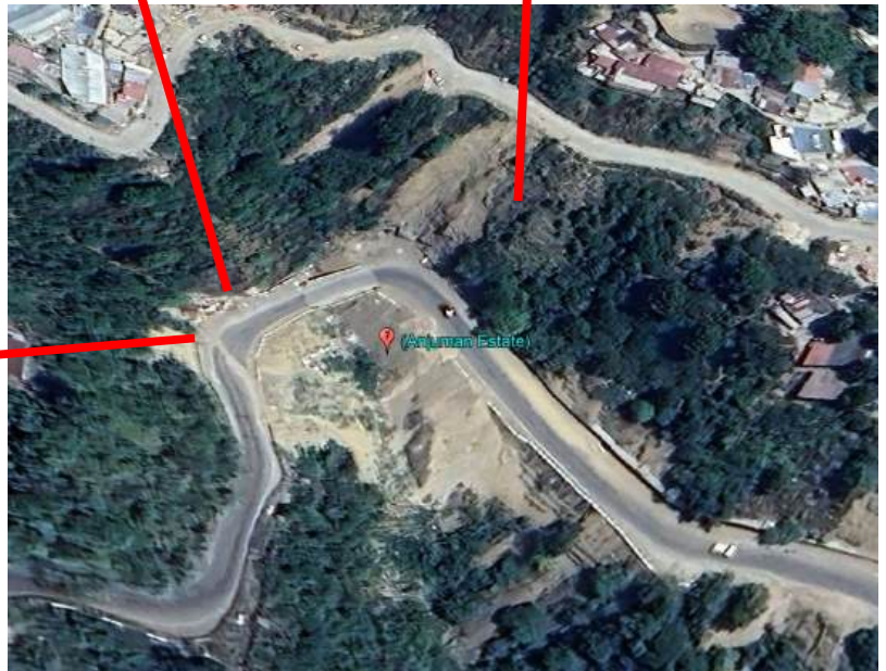
Figure 11 exhibiting the conditions of slope at Site 7
