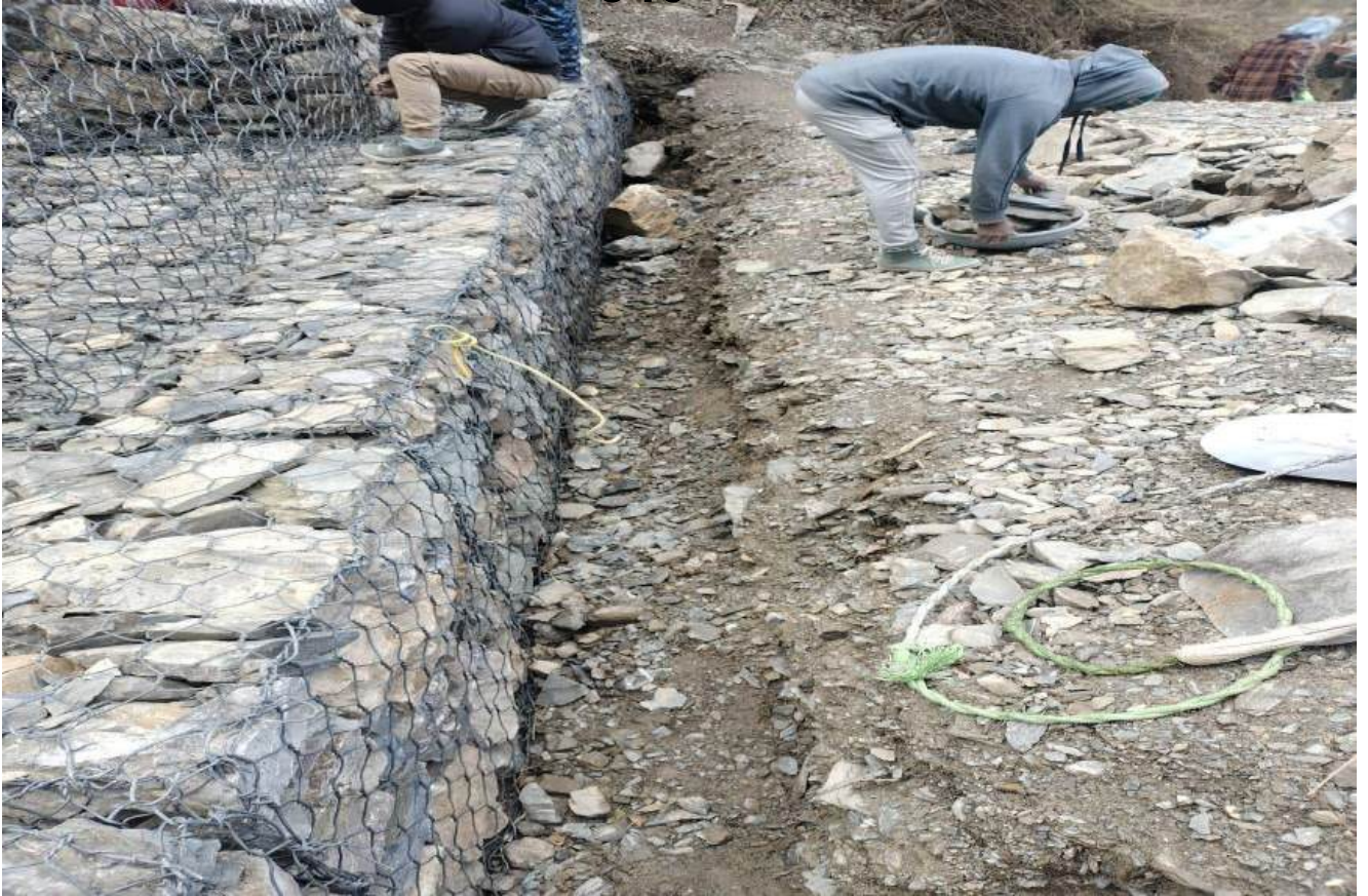
Installation of Gabions at Muck dumping site
