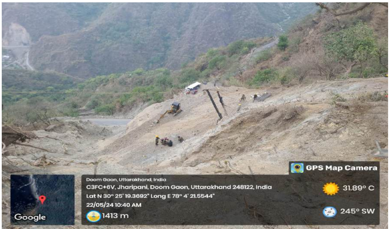
Scaling of Overburden & Making of Benches
